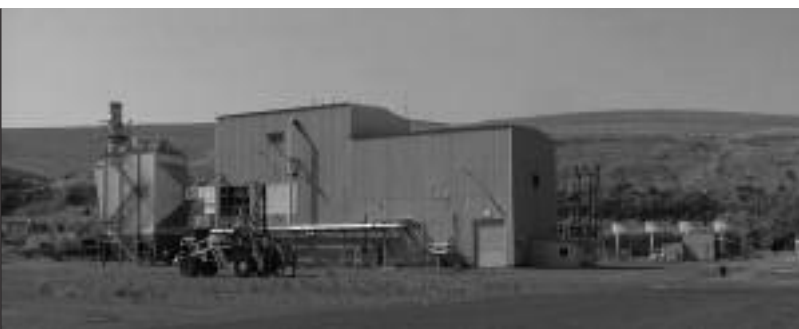
Heppner Generating Plant
