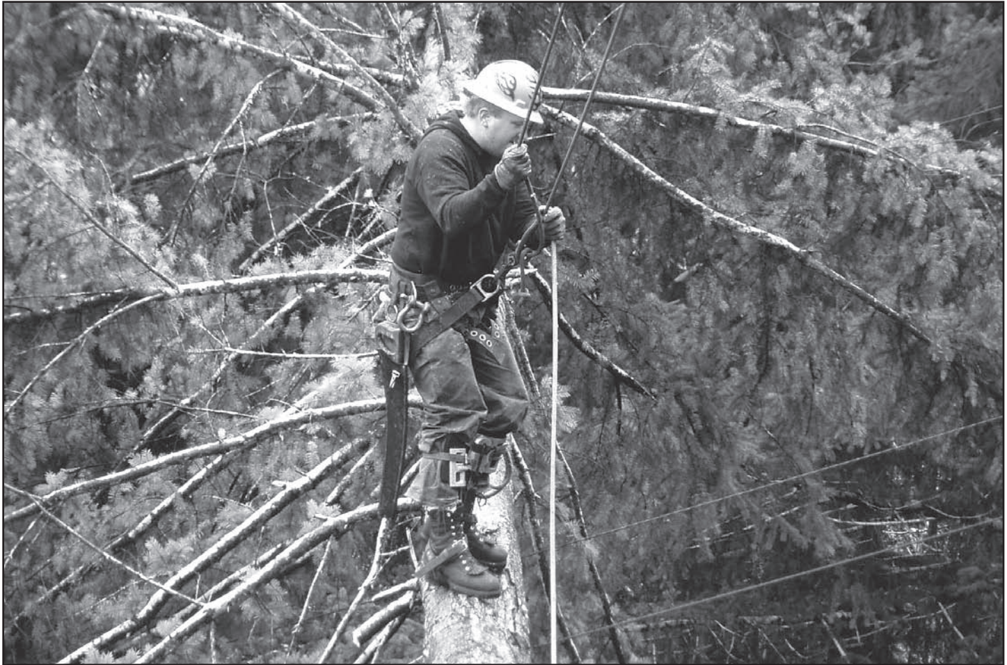
Justin Glasgow, foreman of Utility Tree Service, puts a harness on a tree uprooted by high winds during a November storm in Oregon's Willamette Valley. The tree is propped up by utility lines below it. Opposite page , trees take down a line in the Kings Valley area, west of Philomath, Oregon. Photos courtesy of Consumers Power, Inc.
